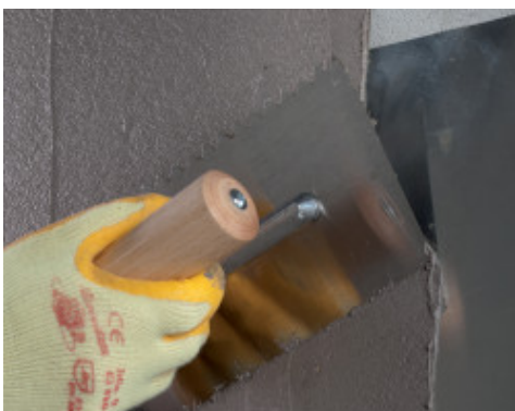
Skim coating and protection of Mapeshield E with Mapelastic Guard Zero applied by trowel
