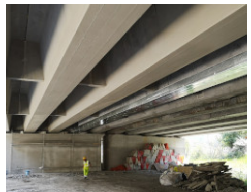
Beams protected with Mapeshield E and Mapelastic Guard Zero
