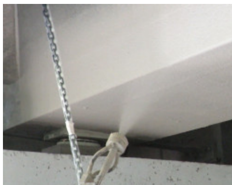
Skim coating and protection of Mapeshield E with Mapelastic Guard Zero applied by spray
